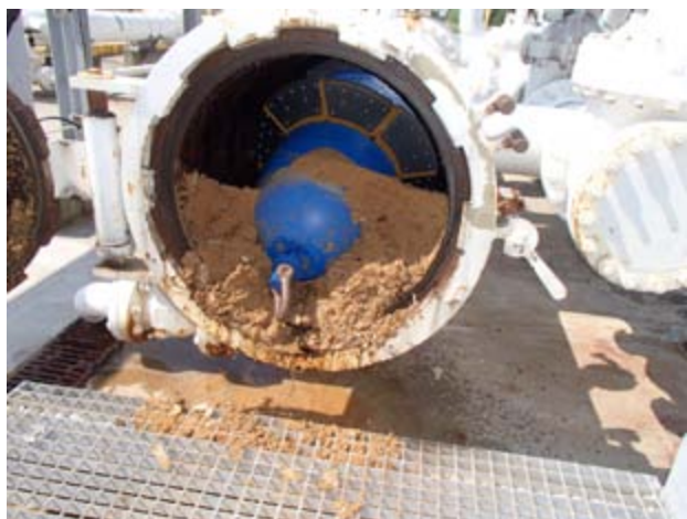
Picture showing retrieval of 24" MCT flushing forward powdered scale
