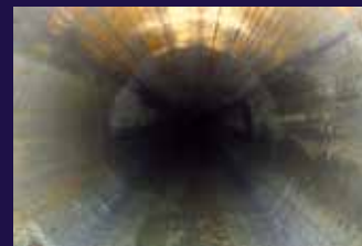
DN200 WATER COOLING LINE
