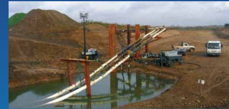
6" OXYGEN PIPELINE (CLEANING, TESTING, DEWATERING AND DRYING)
