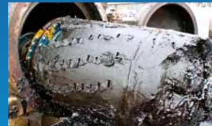
20" CRUDE OIL EXPORT PIPELINE
