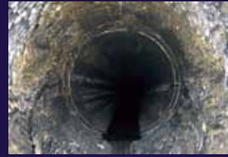
DN250 SLUDGE WATER LINE
