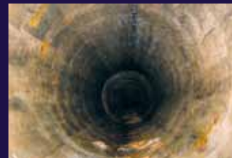
DN150 DRINKING WATER LINE
