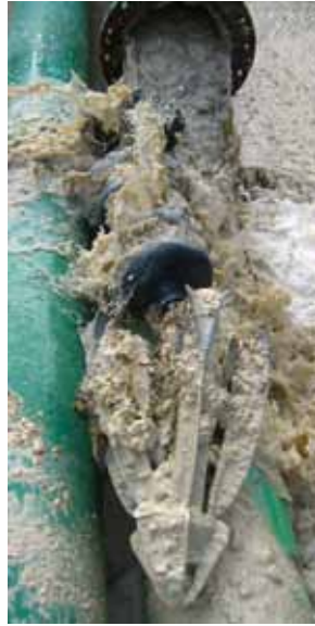
16" LATEX PRODUCTION PIPELINE
