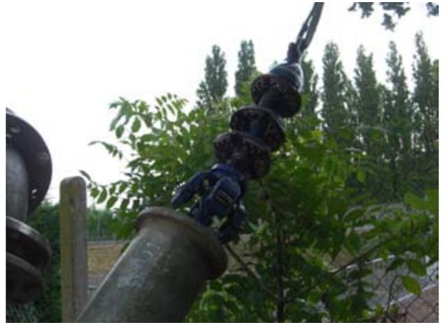
*Pulling out a 6" mechanical cleaning tool*
